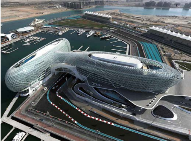
Viceroy Hotel Yas Island F1 Circuit (Abu Dhabi, United Arab Emirates)
